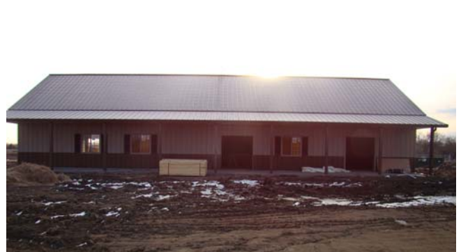
Training building after walls...
